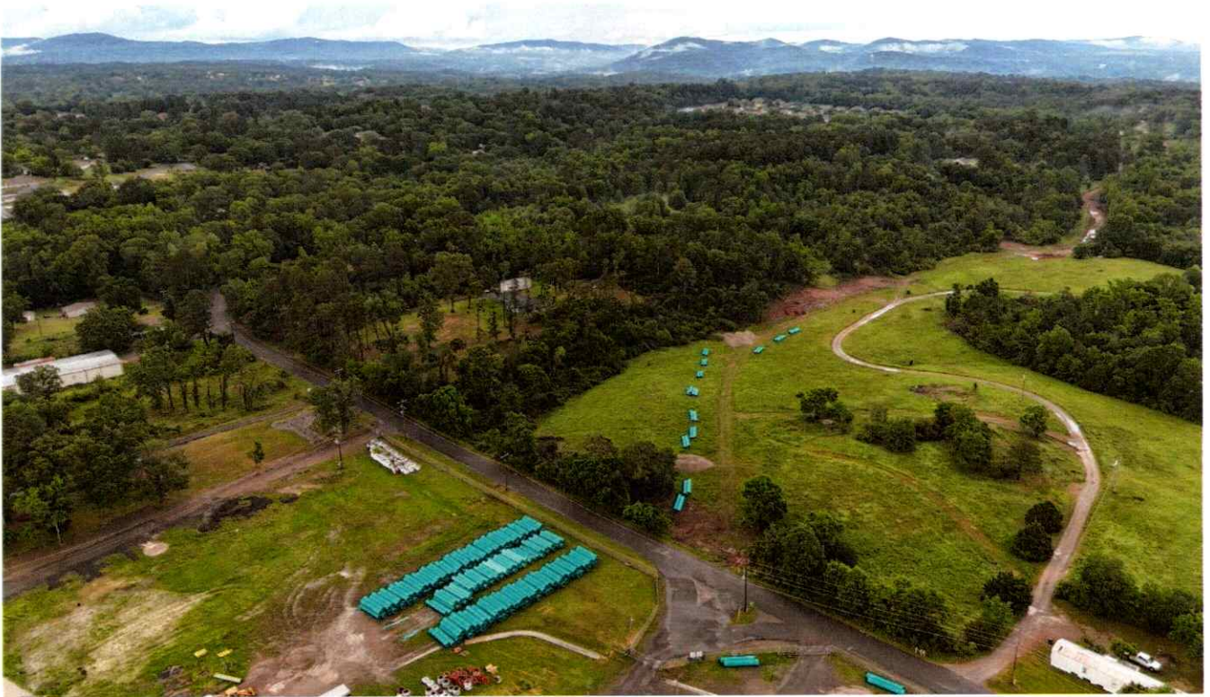
Material staging area near Hot Springs Compost Facility
