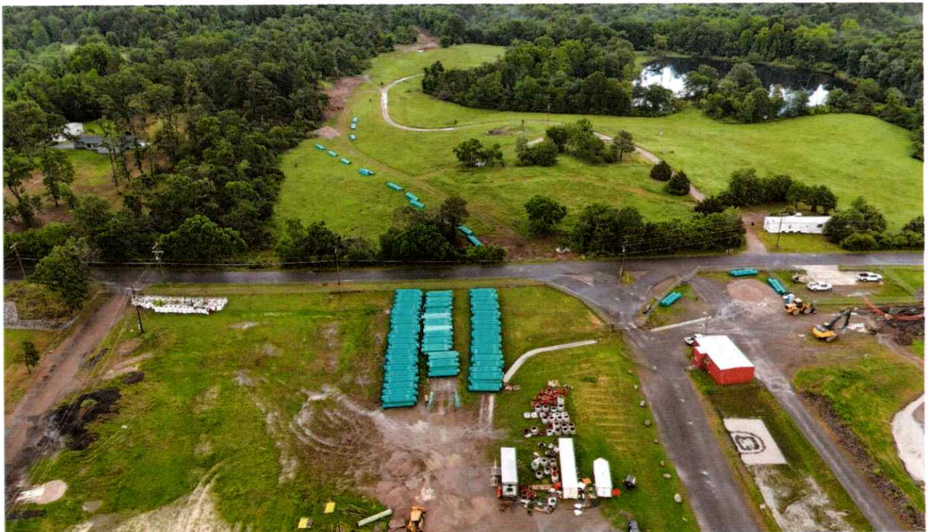
Force main pipe laid out for installation
