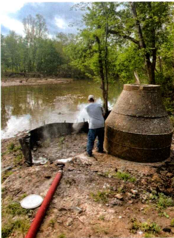
MH 1748 During cleanup – 4/12/25
