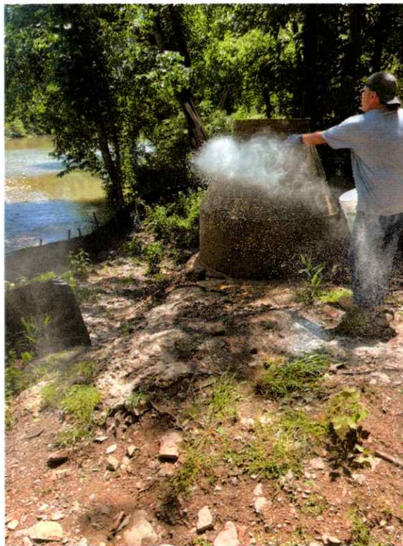
MH 1748 During cleanup - 5/1/25
