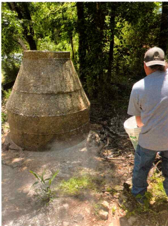
MH 1748 During cleanup - 5/1/25
