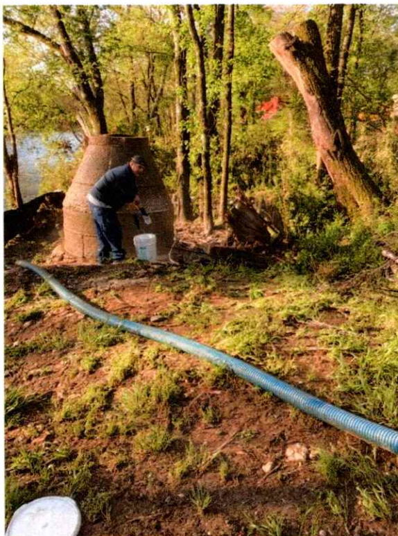
MH 1748 During cleanup 4/8/25
