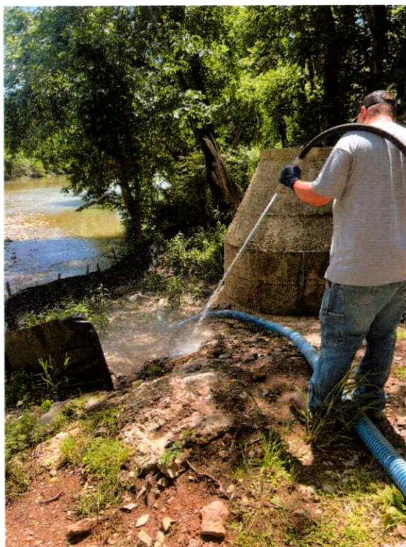
MH 1748 During cleanup - 5/1/25
