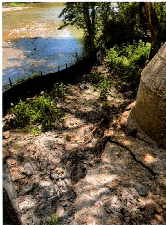
MH 1748 After cleanup – 5/1/25
