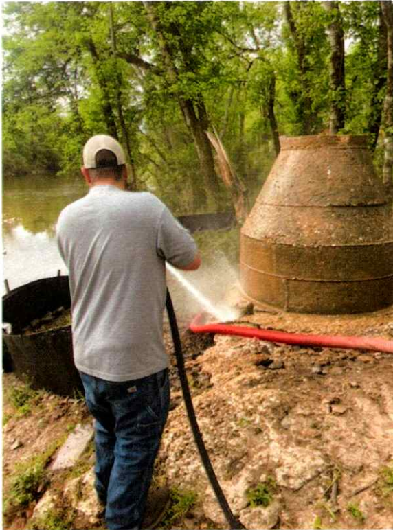
MH 1748 During cleanup – 4/12/25
